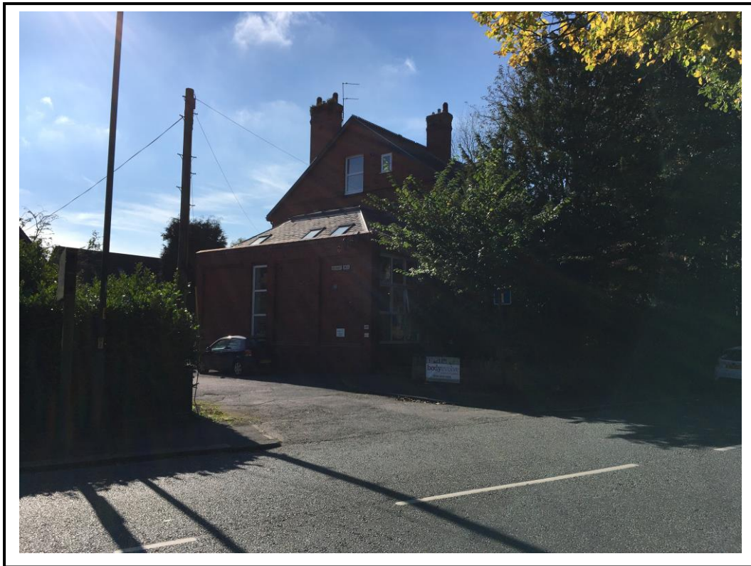
View from Stockport Road
